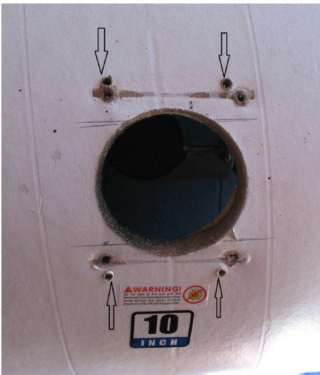
New Holes Drilled
