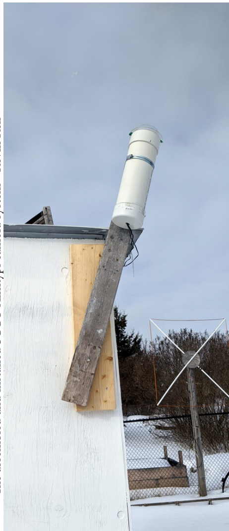
The assembled and installed SCGO Allskypi camera system - Kevin Kell
