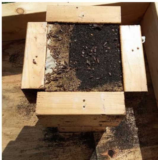
The sand filled interior of the pier.. With free earwigs!
