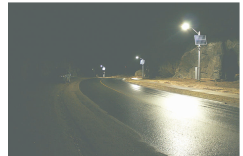
The Forbes’s Hill Rd road towards Lion’s Lookout has modern white LED lighting that overwhelms the visibility provided by car headlights! The LED luminaires have the relatively standard flat-panel of LEDs but they are also tilted up—presumably to illuminate the vertical rock face beside the road (?).
