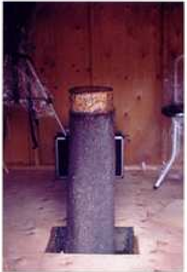
This is a pier for mounting a telescope inside the Gagnons' observatory.
