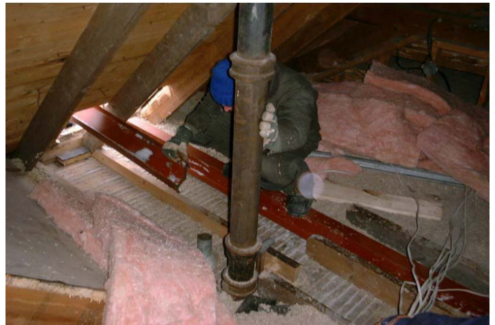
With the first beam in place, the second beam is being carefully moved in. At 400 pounds apiece this takes
