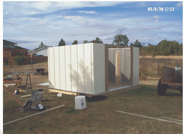
Walls assembled (doors come later)...
